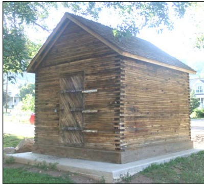
Exterior of Palmer Lake Jail today
